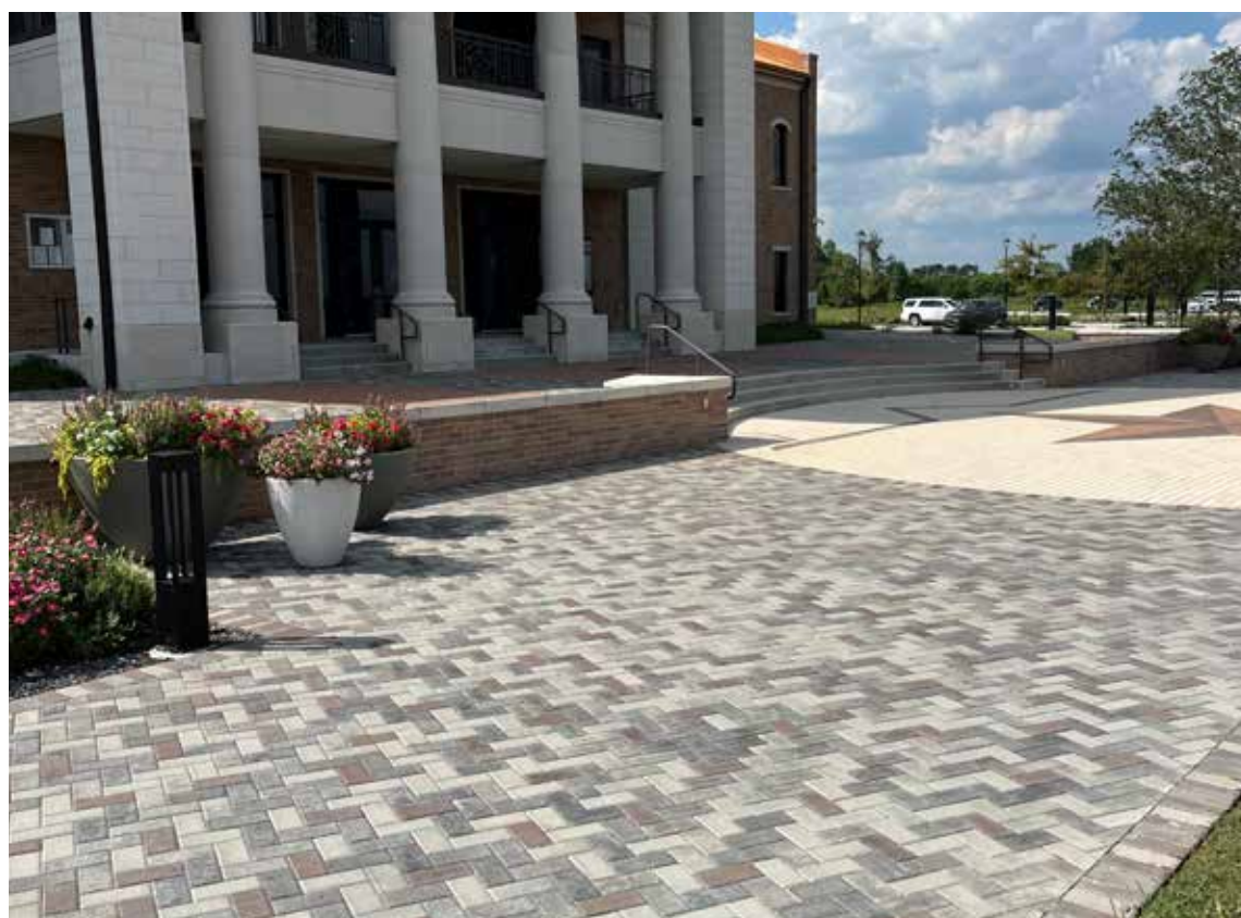
MONT BELVIEU CITY HALL - Mont Belvieu, TX Products & Colors: Holland Stone in Antique Pewter, Antique Terra Cotta, Dark Brown, Limestone, Pewter and River Red Finishes: Standard Architect: BRW Architects Installer: Paveloc Plus
